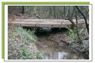
Bridgemats provide a good alternative for temporary stream crossings with minimal impacts to water quality.
